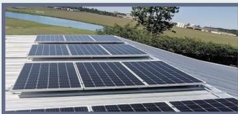
Two photovoltaic systems at NAVWPNSTA-SB have been offline for several years due to maintenance funding issues. The UESC project will replace inverters to get these systems up and running again. This project supports **Resiliency** by lessening grid dependence for electricity.
