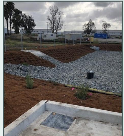
**Storm water retention basin built as part of the MARFORRES Reserve Center LID construction project.**
